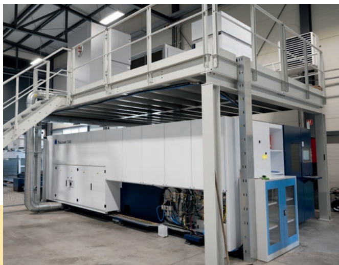
New laser machine from Trumpf at the Rozvadov (CZ) site
